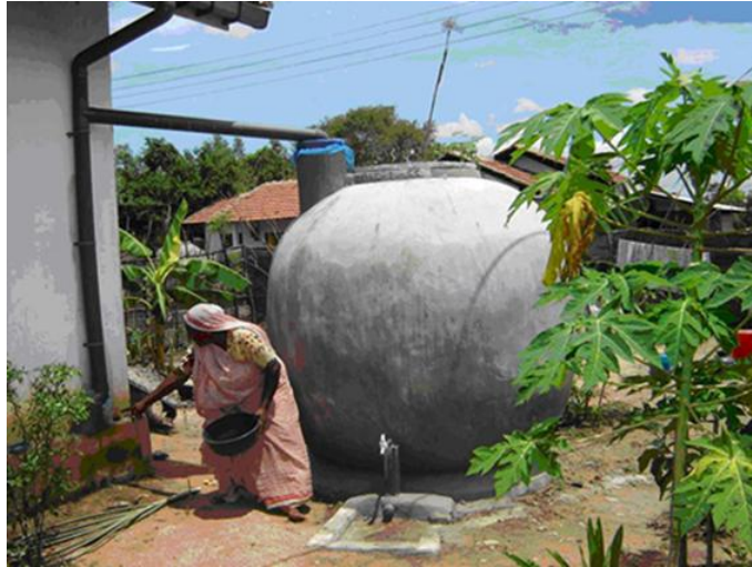
Figure 5 - Rain Water Harvesting Tank
